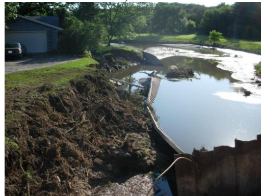
Photo Set 1: Examples of damage to Babbling Brook banks after June 21, 2009 storm.
